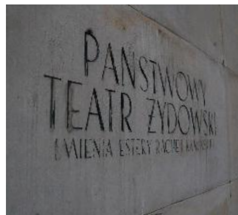
EXISTING STONE CLADDING
